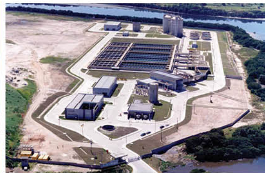
Allegria WWTP, Brazil
