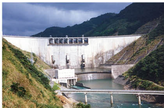
Feitsui Dam, Taiwan
